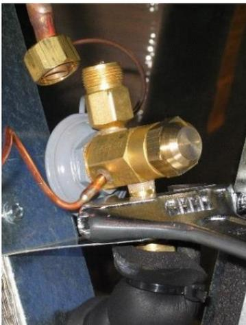
**Figure 9. Attaching TXV to Distributor**
