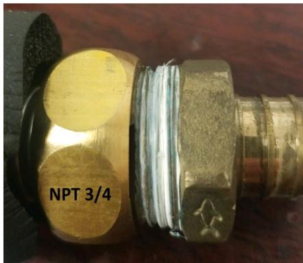
Bellows NPT  $\frac{3}{4}$  to fitting connection
